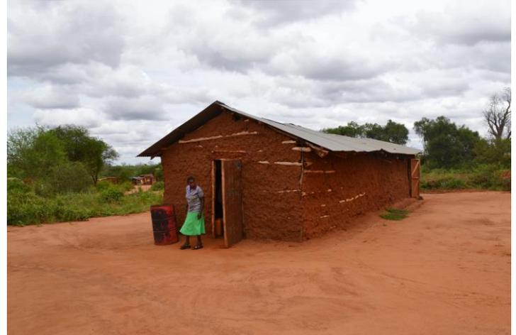
The church here is a small mud building about 15x30. The walls are red mud packed into a lattice of sticks with the ever-present corrugated iron roof. Dirt floor, no windows, and a makeshift door – this is not your standard, everyday church like we would expect in America. This is the evidence of desperate faith and a desire to worship God where it is not convenient.
